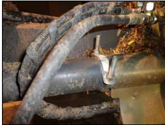
FIGURE 10. Large Muffler Clamp Installed
