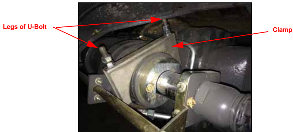
FIGURE 4. Muffler Clamp Installed on Steering Cylinder Barrel
