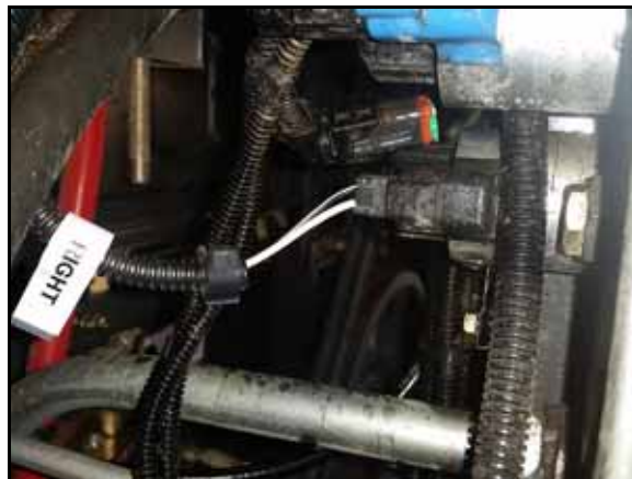
FIGURE 14. RIGHT Valve Harness Connector Installed
